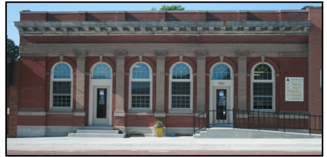
Renovated AAM office in Milford, NE.
