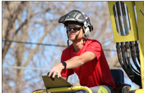
Brandon working grapplesaw/crane controls
