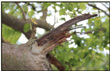
Figure 3: In branch failure from high winds, the remaining splinters will typically point upwards. When a failure occurs from loading or no wind, the splinters will typically point downwards. Branch fractures and stubs create long-term entry points for harmful organisms and often lead to the development of wetwood. For this type of wound, Natural Target Pruning to the branch bark collar can eliminate the stub, encourage the development of woundwood and potentially close and encapsulate harmful organisms.
