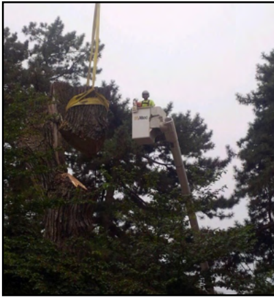
Tree removal using a bucket.
